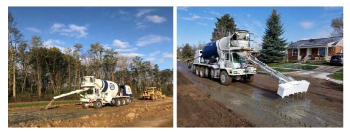
Cement slurry is spread from a ready mixed concrete truck. Photos courtesy of Scott Hall, Sagamore Ready Mix, (left) and Dr. Spencer Guthrie, BYU.
