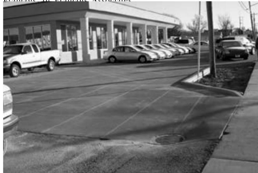
Above: Large columns, added overhang, and a concrete parking lot contributed to the exterior appearance of the facility. A combination of UTW and transition slabs converted an unsightly asphalt surface to a well-drained attractive concrete surface.
