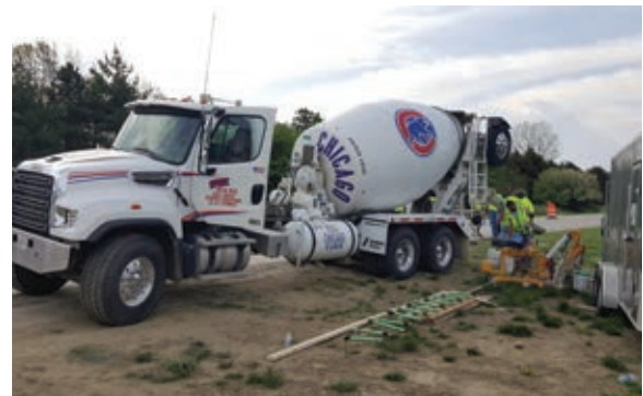
Sport Redi-Mix in Champaign, Illinois, delivers concrete in their Chicago Cubs mixer. This highway project was completed for IDOT.
