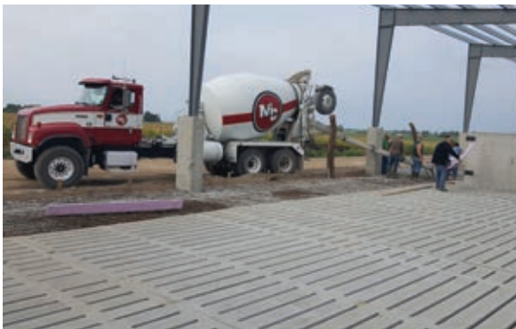
Mid-Illinois Concrete provides concrete for a hog confinement project. The concrete was dispatched from their plant in Effingham, Illinois.
