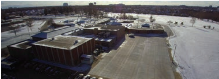
Concrete overlay project at Glenn Westlake Middle School in Lombard. Concrete supplied by Elmhurst Chicago Stone.
