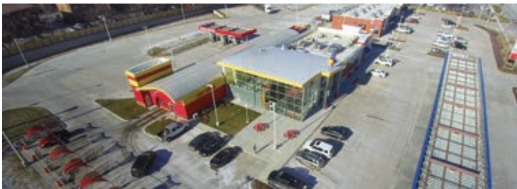
Ricky Rockets Gas Station project in Midlothian. Concrete supplied by Welsch Ready Mix of Oak Forrest and placed by Abbey Paving.
