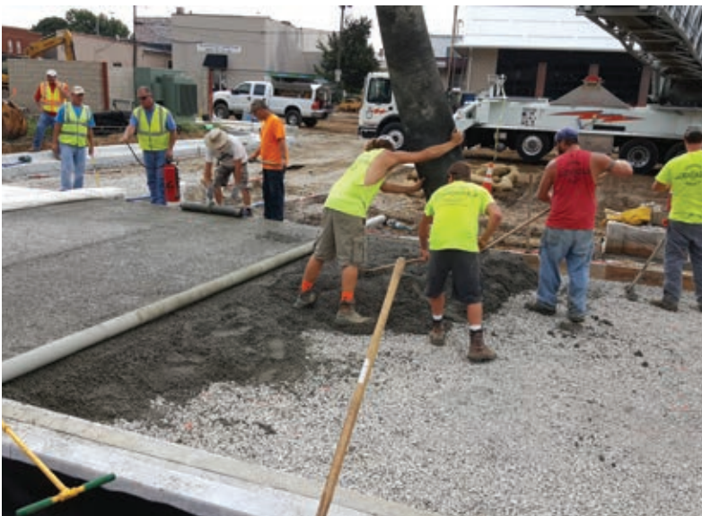
Aupperle Construction is placing pervious concrete for a parking lot in Morton, Illinois. VCNA Prairie's Central Illinois Division supplied the concrete.
