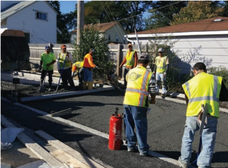
R W Dunteman placed pervious concrete for an alley project in Westmont, Illinois.
