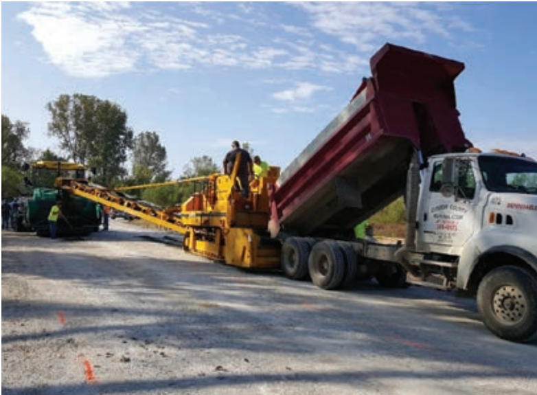
Quad-County Ready Mix supplies 3,200 cubic yards of roller compacted concrete for a road in St. Claire County, Illinois. They delivered it in dump trucks to speed up the paving process.
