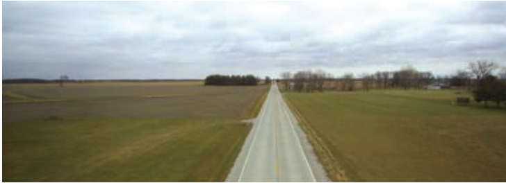
County road project in Oconee township. Concrete supplied by MBI Construction of Effingham.
