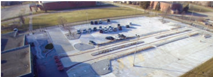
Concrete overlay project at Altamont Company in Rantoul. Concrete supplied by Blager Concrete Company of Urbana and placed by I C Contracting.
