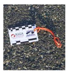
To ensure adequate bond between the concrete and the asphalt overlay, the surface is power-broomed and air-blasted. This leaves a clean surface with adequate macrotexture to promote bond.
