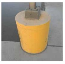
Expansion material around the light standards allows for differential vertical movement due to freezing and thawing and prevents inadvertent adhesion between the parking lot surface and the standard. Improper handling of this can lead to problems.
