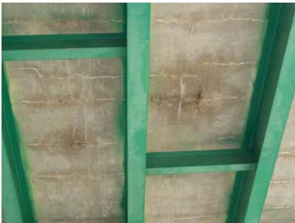
*Cracks as seen from the underside of a bridge*
