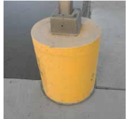
Expansion material around the light standards allows for differential vertical movement due to freezing and thawing and prevents inadvertent adhesion between the parking lot surface and the standard. Improper handling of this can lead to problems.
