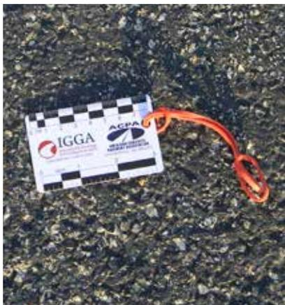
To ensure adequate bond between the concrete and the asphalt overlay, the surface is power-broomed and air-blasted. This leaves a clean surface with adequate macrotexture to promote bond.
