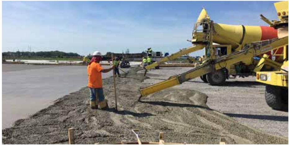
Rock River Ready Mix delivered concrete to a Deer Creek ComEd project that required anywhere from 22 to 140 cubic yards per drilled shaft.
